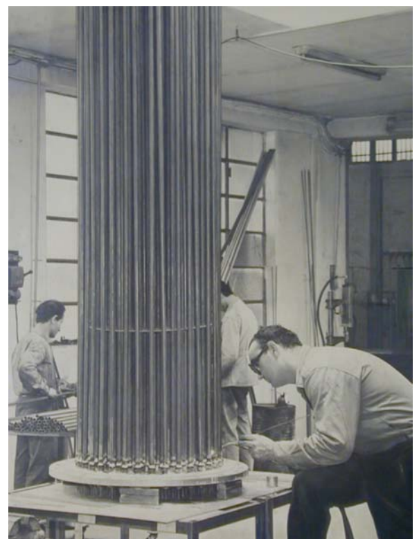
Braze Welding of the first flange-mounted heater Year 1967
